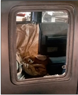
Installed weather seals
